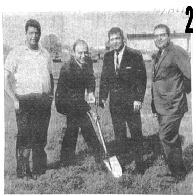
PENDLETON CEREMONY —The first spadeful of dirt was dug Monday for the new Pendleton Town Building. Participants are, left to right, Albert Virtuoso, of Virtuoso Building Co., Inc., general contractors; Donald D. Lanternier, Building Committee chairman; Raymond A. Beiter, town supervisor; and Charles M. Hall, town engineer.
